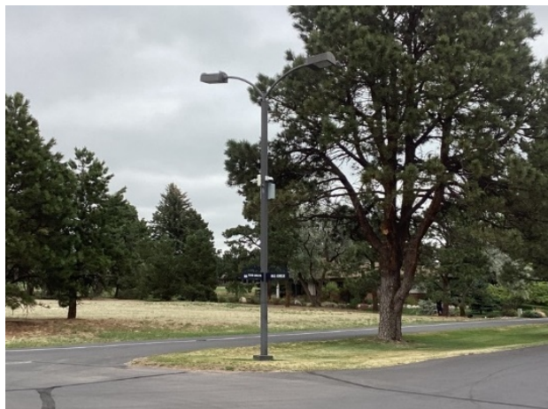
Light pole and fixtures
