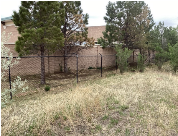
Chain link fence
