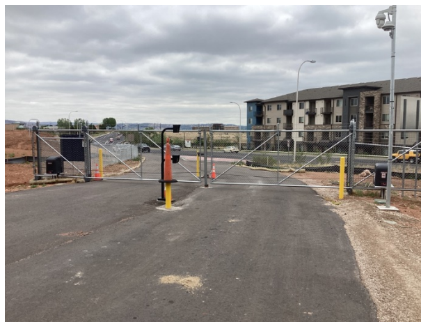
Construction gate entrance
