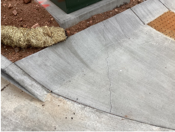
Sidewalk cracks
