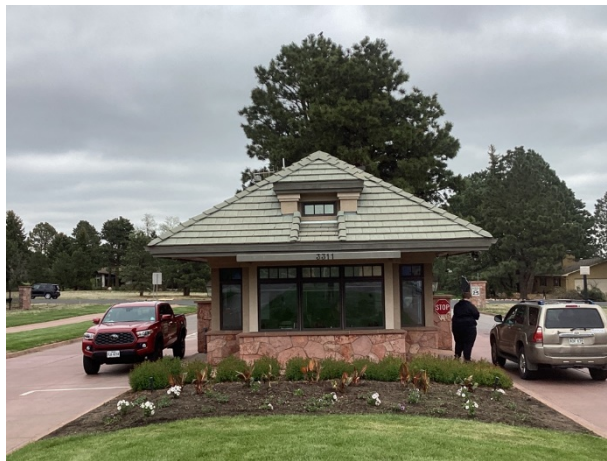
Guard house overview
