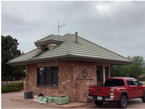
Gate house concrete tile roof
