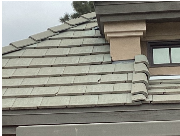
Damaged tiles
