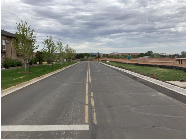
Asphalt pavement street overview
