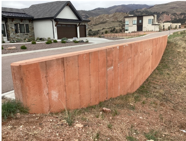
Concrete retaining wall
