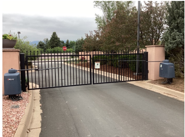
Steel gates at west residential entrance
